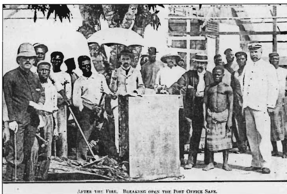
Figure 3 After the Fire. Breaking open the Post Office safe (from Ref. 1)
